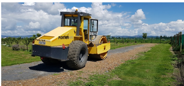
Past pupil James Barker rolling the new entrance way for the development project next to the Hayward Farm.
