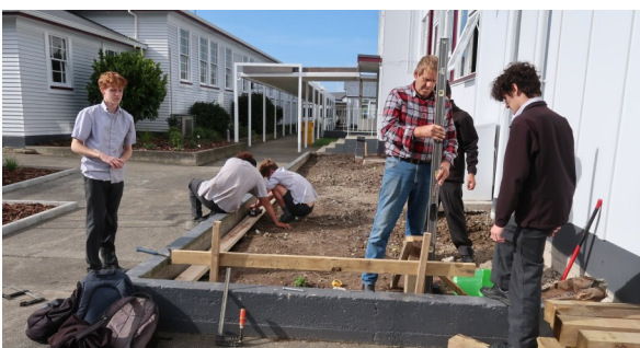
Year 13 BCT building a deck
